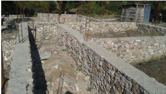
SCHOOL CONSTRUCTION GETS UNDERWAY
