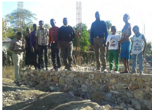
FATHER NOÉ BERNIER CHECKS ON PROGRESS AT THE PACASSE SCHOOL SITE
